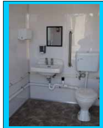
ADA Lavatory Stall
