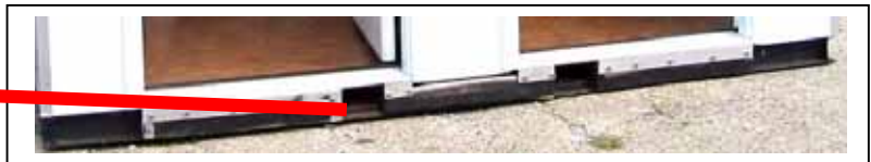
Fig. 2 - Tine Ports (Steel Frame)
