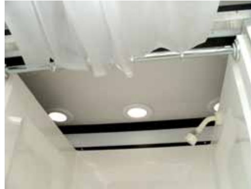
Rear Ceiling/Skylights Shower Head
