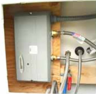
Tank-less Hot Water Requires 220 V (US) 206 (UK)
