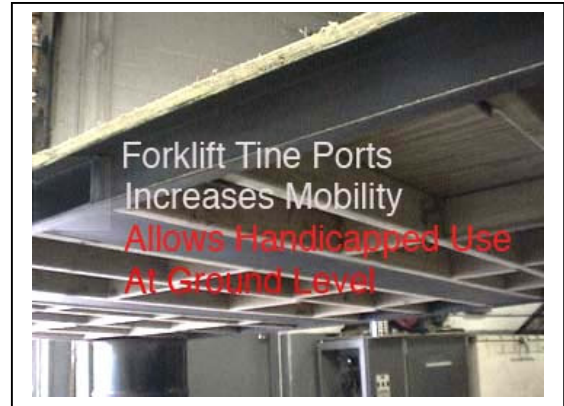
View of Frame Under Section
